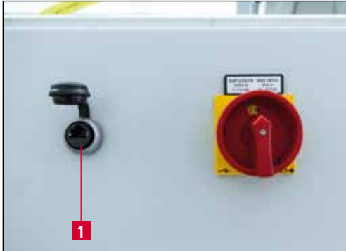
Figure 8-14 Power supply connection
