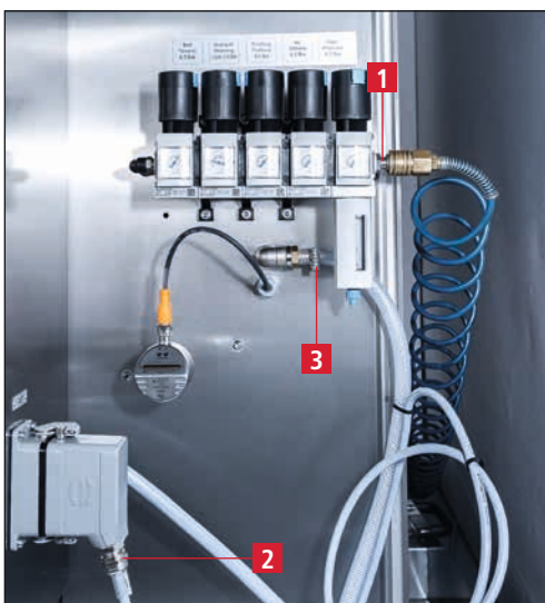
Figure 6-2 Compressed air connection
