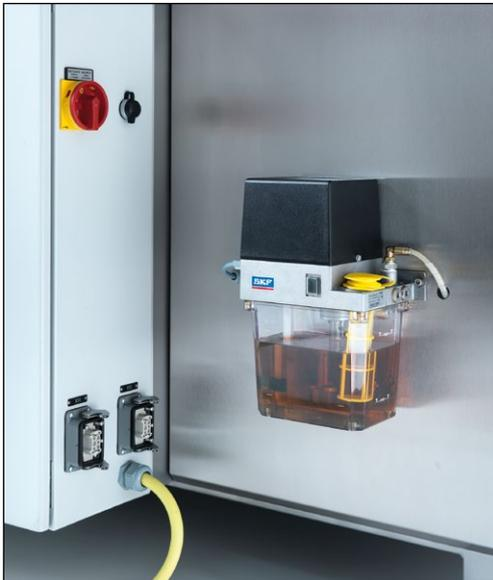
Figure 9-1 Lubrification centrale
